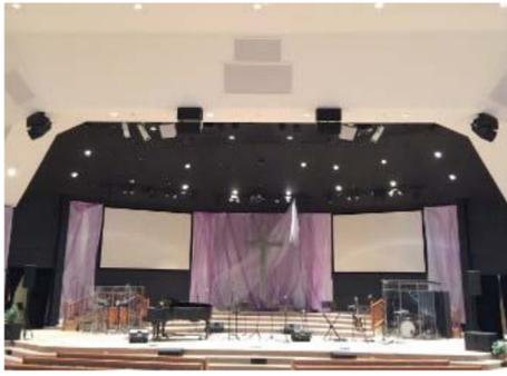
A pair of **dsPEC226AN** DSP processors provide loudspeaker management, delay and equalization. The church's existing under-balcony loudspeakers were reused, but the full-range performance of the I SERIES allowed them to turn off the existing subwoofers.
